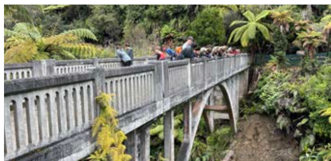
Bridge to Nowhere Walk on Day 2 of the Whanganui River Journey.
